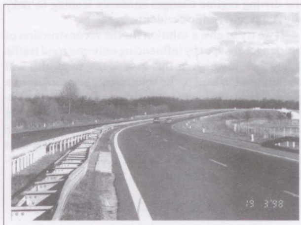
Photo 1 - Condition of the considered curve before reconstruction
