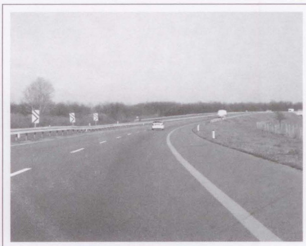
Photo 2 - Condition of the considered curve after reconstruction
