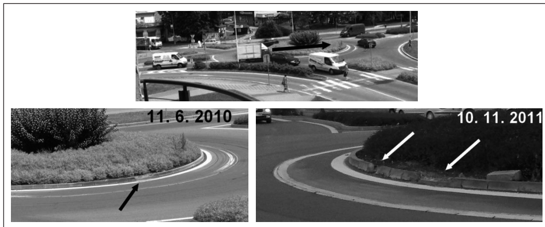
Figure 6 - Photographs of conflict situation 4f_{p2} (roundabout No. 15 – see Table 1) and details of damaged curb of the central island (the same place at an interval of approx 1.5 years)
