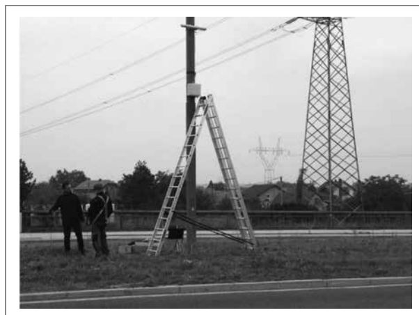
Installing the radar to verify speed profiles
