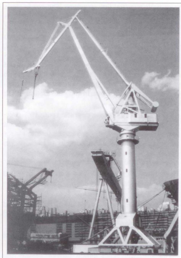
Figure 4 - The slewing port jib crane in the 3. Maj shipyard, Rijeka, Croatia
