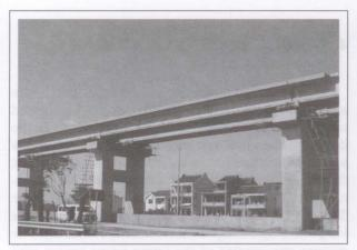
Figure 6 - Hybrid guideway girders along the track
